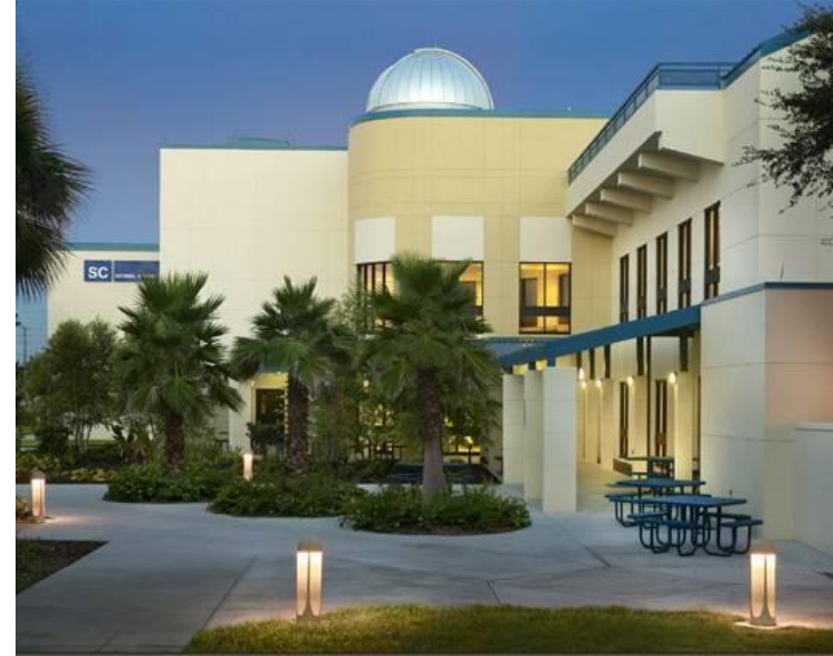
Natural Science Building Blue Metal Roofs
